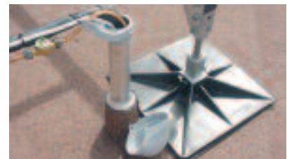
3. Use knock holes to take pipes/cables through.
