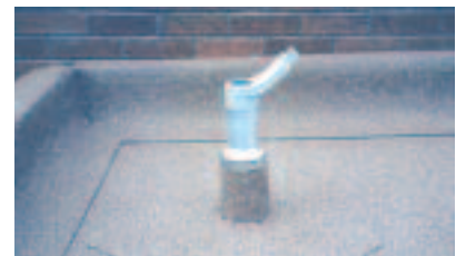
2. Waterproof the base and upstand.
