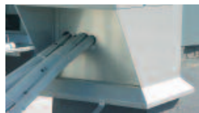
4. Cut pull-out panel to pipe work.
