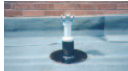
1. Mechanically fix the base unit to the deck.
