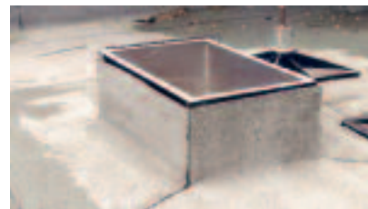
2. Waterproof the base and upstand.
