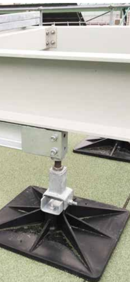
HOT DIP GALVANISED SUPPORT FRAME
