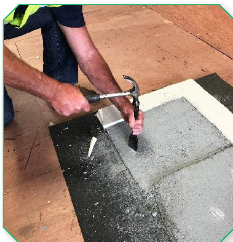
Within approximately 30 minutes from mixing the Monoscreed passed chisel & hammer test.
