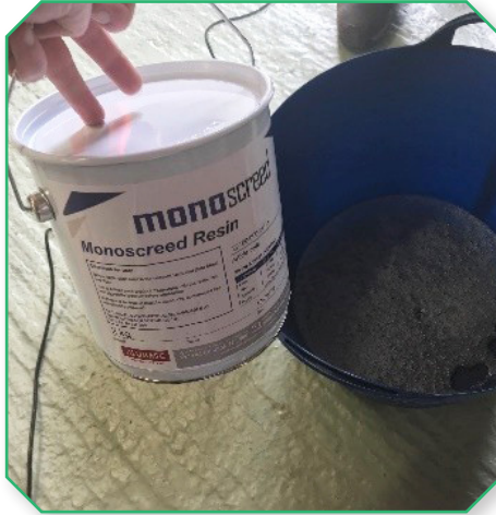
Pour into bucket 2kg of Monoscreed resin.
