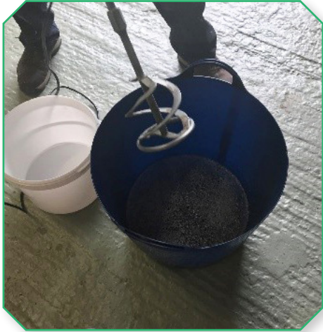
Use large bucket for mixing. Power drill with paddle to be used for mixing.
