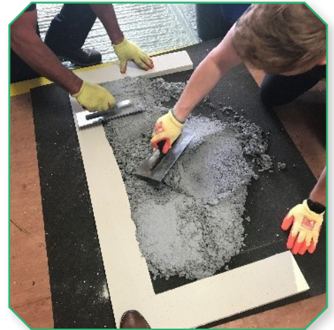
Use trowel to tamp & level the Monoscreed.
