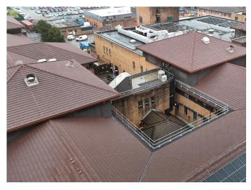
Airtile is BBA approved, ISO 14001 certified, and manufactured using ISO 9001 approved materials. It is Fire resistant to AA classification: equal to traditional roof tiles and slates. Importantly, the system offers quick installation times, which were key for the Princess of Wales roof in order to get the hospital back up and running as normal within the most efficient timescale.
